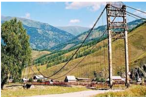
Bridge under Katun river near Tungur village
